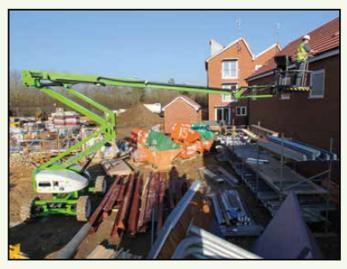
The tough, impact-resistant composite base and larger cross-section steel rails of the HR17 4x4's **ToughCage** give extra strength and durability and the multi award winning **SiOPS**® provides additional operator protection.
